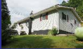
913 St. Hwy 1661, Grayson $85,000 3 BR, 1 BA ranch w/new metal roof, dishwasher, newer hot water heater, HW floors under carpet plus more. Norma Mullins 922-4552
