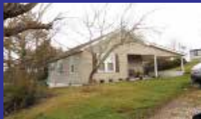
114 E. Fourth St., Grayson $55,000 2 BR, 1 BA, new dimensional shingled roof, vinyl siding, windows, cabinets & BA fixtures. Norma Mullins 922-4552
