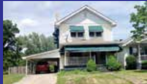
3251 Short St. $65,000 2 BR, 2 BA, lg 2 story, lg FR, new roof. Nice for 1 st time home buyer or rental. Denise Cumpton 694-3137
