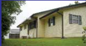
1211 Raceland Ave. $68,000 3 BR, 1 BA nice ranch. One car garage, roof shingles & HVAC replaced in 2015. Location qualifies for 100% financing. John Daniels 606-922-7633, Johnda McGuire 606-615-1927
