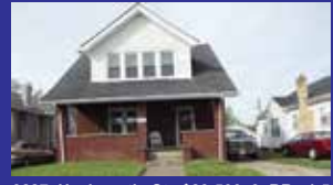
3227 Hackworth St. $89,500 3 BR, 1.5 BA, 1.5 story, 1,300 sq.ft., fully equipped kitchen & lg DR. Newer heat & air plus windows. Laundry & half BA on main. Denise Cumpton 694-3137
