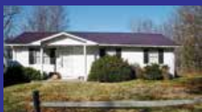
4123 Marsh Hill Dr., Catlettsburg $60,000 4-plex. 3 single family dwellings on one lot. Built for rental property. Each has new metal roof & more. Brenda Burns 922-4052
