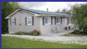
1324 Cantrell St. $78,500 3 BR, 1 BA, vinyl ranch. Cute, clean & cozy. Newer metal roof, vinyl siding, replacement windows, some carpet & paint + more. Brenda Burns 922-4052
