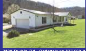
7102 Durbin Rd., Catlettsburg $77,500 3 BR, 2 BA well maintained doublewide on block foundation w/newer metal roof & new furnace. Plus more. Brenda Burns 606-922-4052
