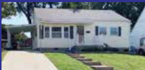
4024 Ferguson Dr. $89,900 2 BR, 1 BA, updated cottage. Updates include exterior doors, shingles, kitchen, flooring, blinds & paint. Outside shutters & landscaping & more. Missi Adkins 606-923-3129, Libby Fugitt 606-571-6401
