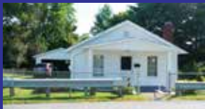
2220 Main St. $49,900 2 BR, 1 BA, cottage that is neat & clean. LR, DR, eat-in kitchen w/gas stove & electric cook top. Side & rear porches, unfin bsmt, det garage. Judy Robinson 606-923-3135
