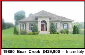
19850 Bear Creek $429,900 - Incredibly beautiful custom built home on 2.5+/- acres with 8 BR including 2 master suites, 3.5 BA featuring an open floor plan w/great room, frpl, granite in kitchen plus underground utilities. Homes was featured in "Street of Dreams." M246724
