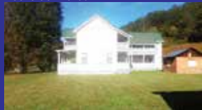
2031 S. Ky 32, Sandy Hook $139,900 3 BR, 1 BA, 70 Acres. 32x66 metal bldg w/ concrete floors & car lift. Newer windows & floor coverings + more. M286325 Jody Mayo 922-4200
