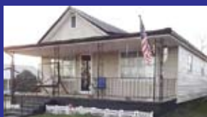
444 4th Ave., Worthington $75,000 2 BR, 1 BA, newer siding, metal roof w/warranty, hot water tank, stainless appliances, 2 car garage, all on corner lot. M65611 Denise Compton 694-3137
