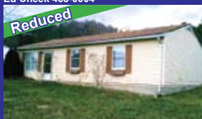
4618 St. Rt. 2, Greenup $35,000 3 BR, 1 BA ranch, great starter home or investment property. Fenced level back yard. M152231 Angela Coovert 571-6296
