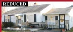
346 Warren Ave. - West
