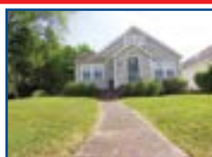
Corner Lot Lots Of Work Done #151399 $84,900
